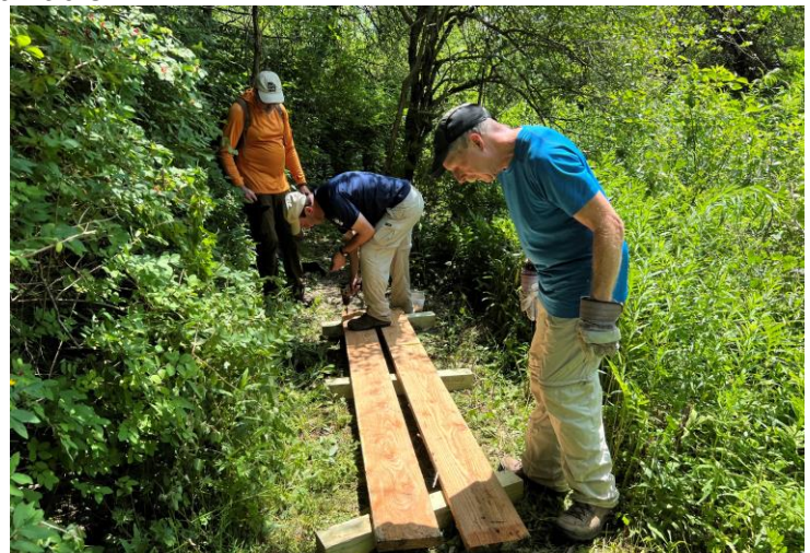
Paul Dobrzynski, Bob Rosati, and Dick Harper assemble a puncheon in Tioughnioga WMA Photo Courtesy Harold Kyle
