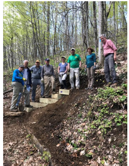
On May 6, chapter members built box steps in Morgan Hill State Forest where rain had washed out a steep section of trail. Photo Courtesy Dick Frio
