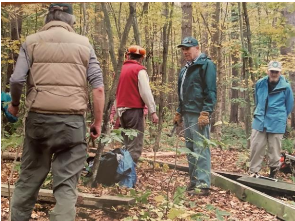
2004 Taylor Valley, removing bridge and reclaiming wood. Bill Brosseau center.
