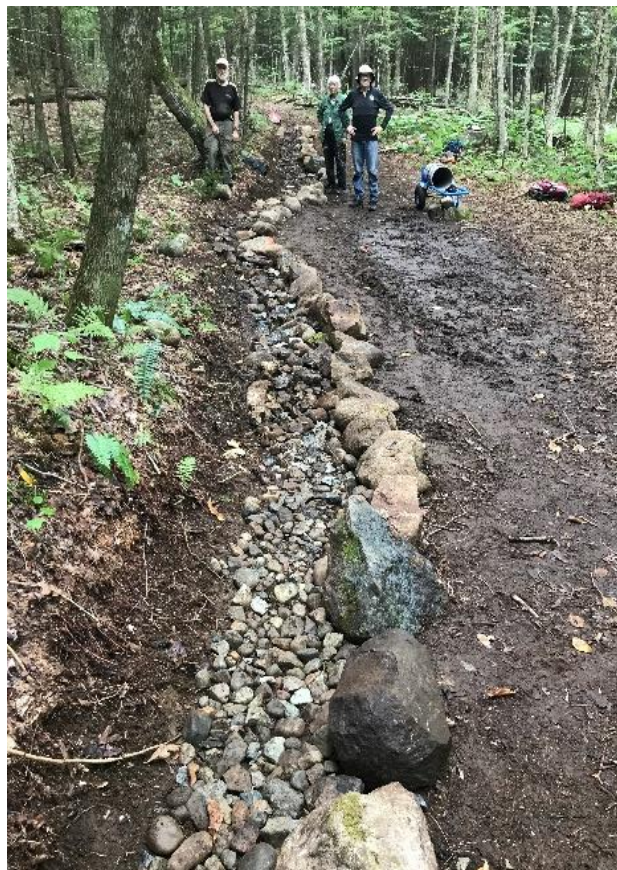
90' turnpike with stone floor ready to be filled with gravel. Steve Hayes, Joan Young, Kevin Moriarity
