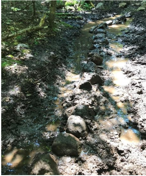
Mudhole in need of turnpike, outer wall in place
