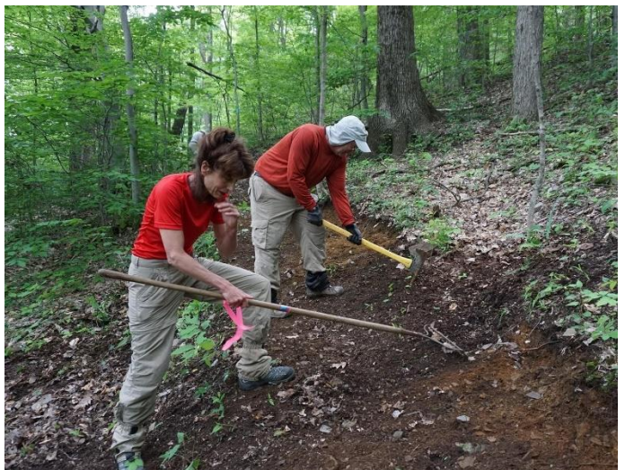
Sandy Manca and Mike Graser benching a trail at Tinker's Falls, June 2. Photo Mike Graser
